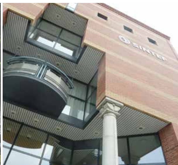
SINTEF Petroleum office
